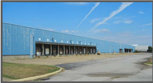
24 Doors on Warehouse A
